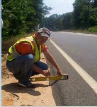
Example of SafetyEdge<sub>SM</sub> after backfill material settles or erodes.
