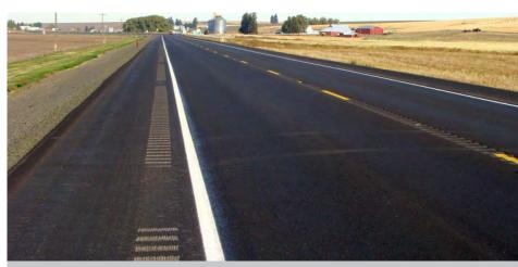
Shoulder rumble strips and center line rumble stripes are installed on this roadway.
